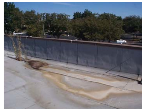
Evidence of water ponding
